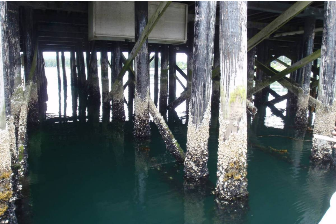
Photograph 4. Typical Bent
