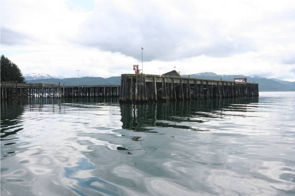
Photograph 1. Overall View of Dock
