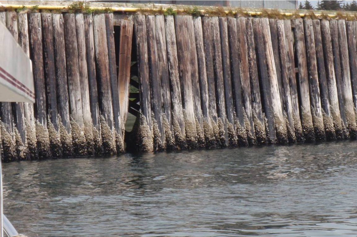
Photograph 14. Wave Screen Missing Pile
