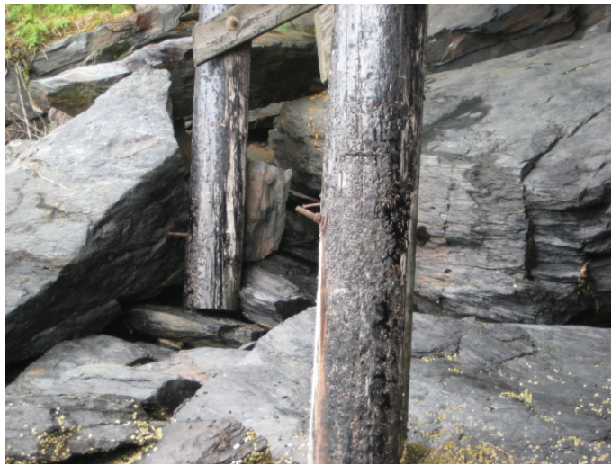
Figure D-4. Unbraced piles on bedrock with bolts indicating missing bracing
