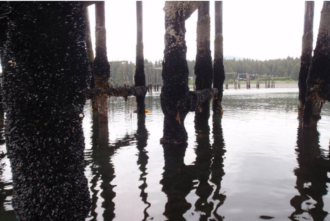
Photograph 10. View Typical Cross Bracing Deterioration
