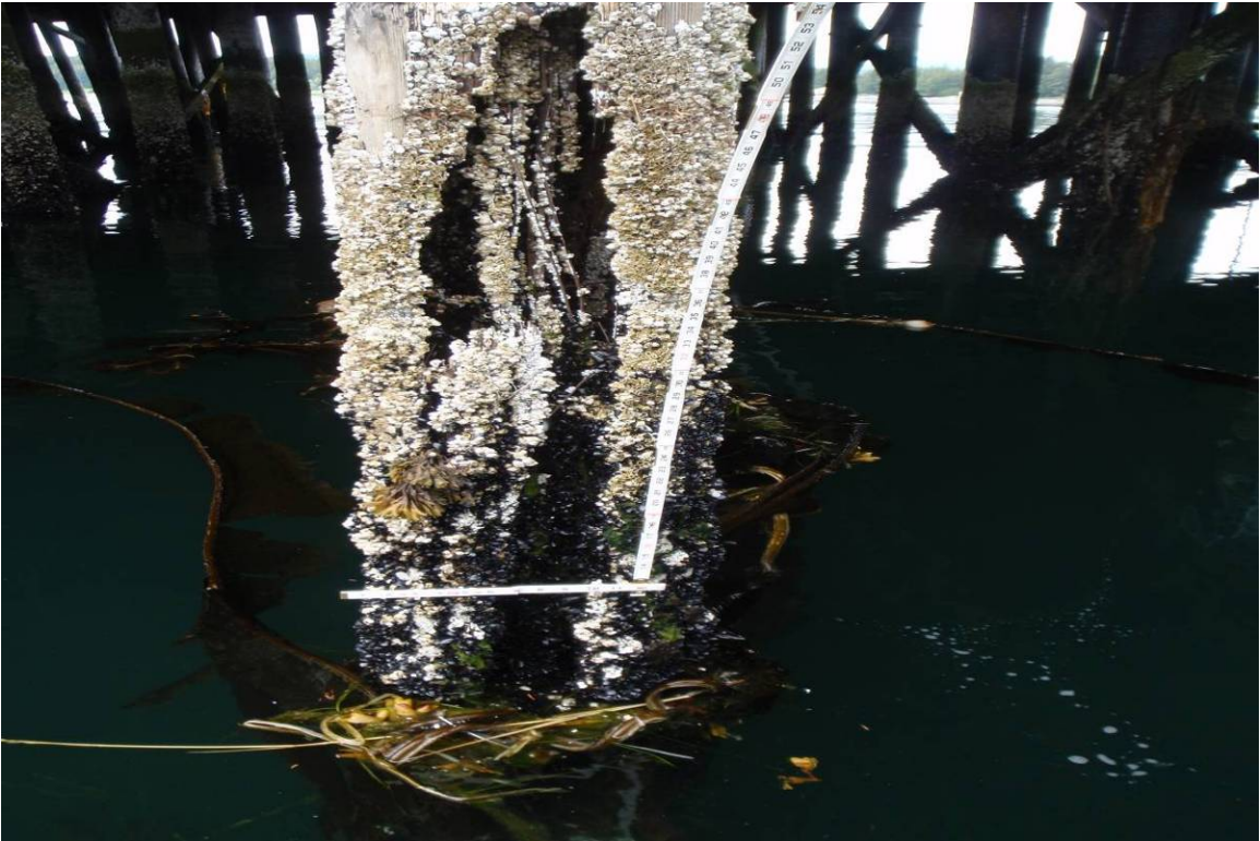
Photograph 11. Pile 35-J, Timber Fender Deterioration
