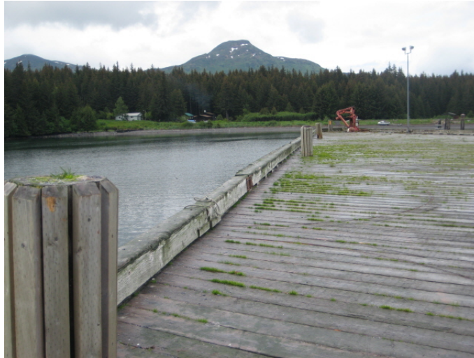
Figure D-11. Typical dock surface with vegetative growth
