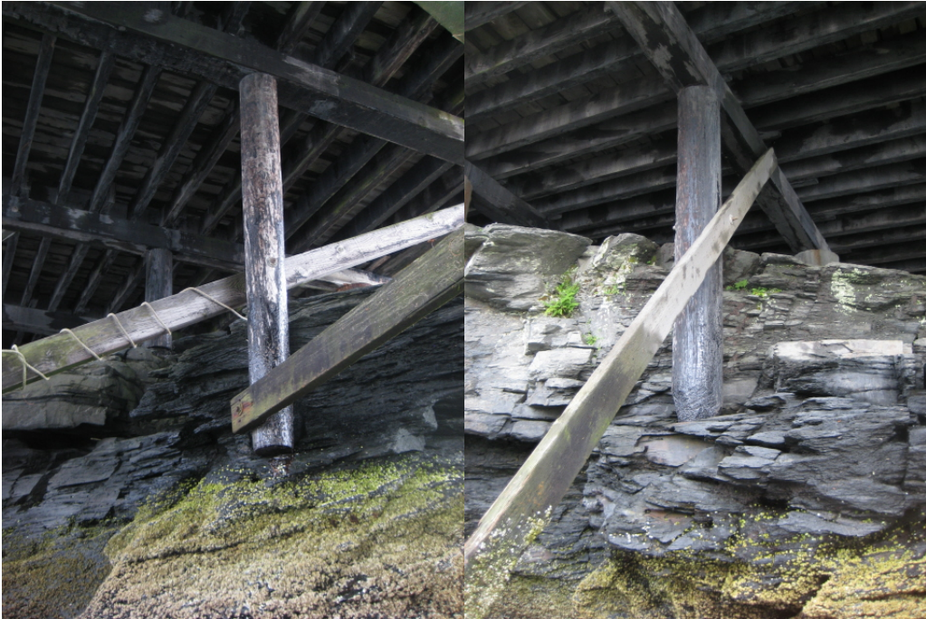
Figure D-3. Unbraced piles on bedrock
