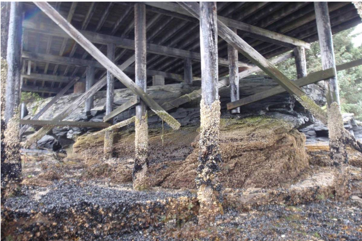
Photograph 6. Bent 7, View of Embankment
