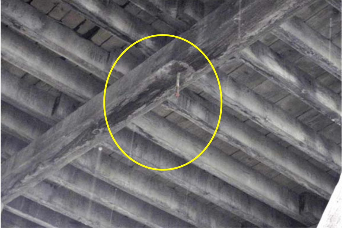
Photograph 9. Bent 10 – Pile C Missing – Cap with Drift Pin
