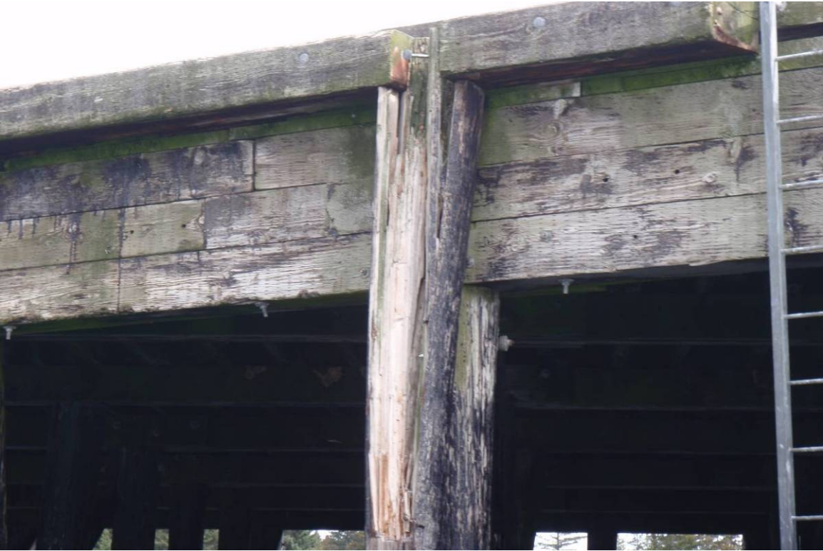
Photograph 12. Timber Fender N Broken
