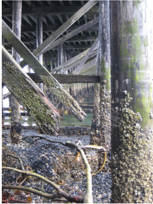
Figure D-5. View underneath causeway
