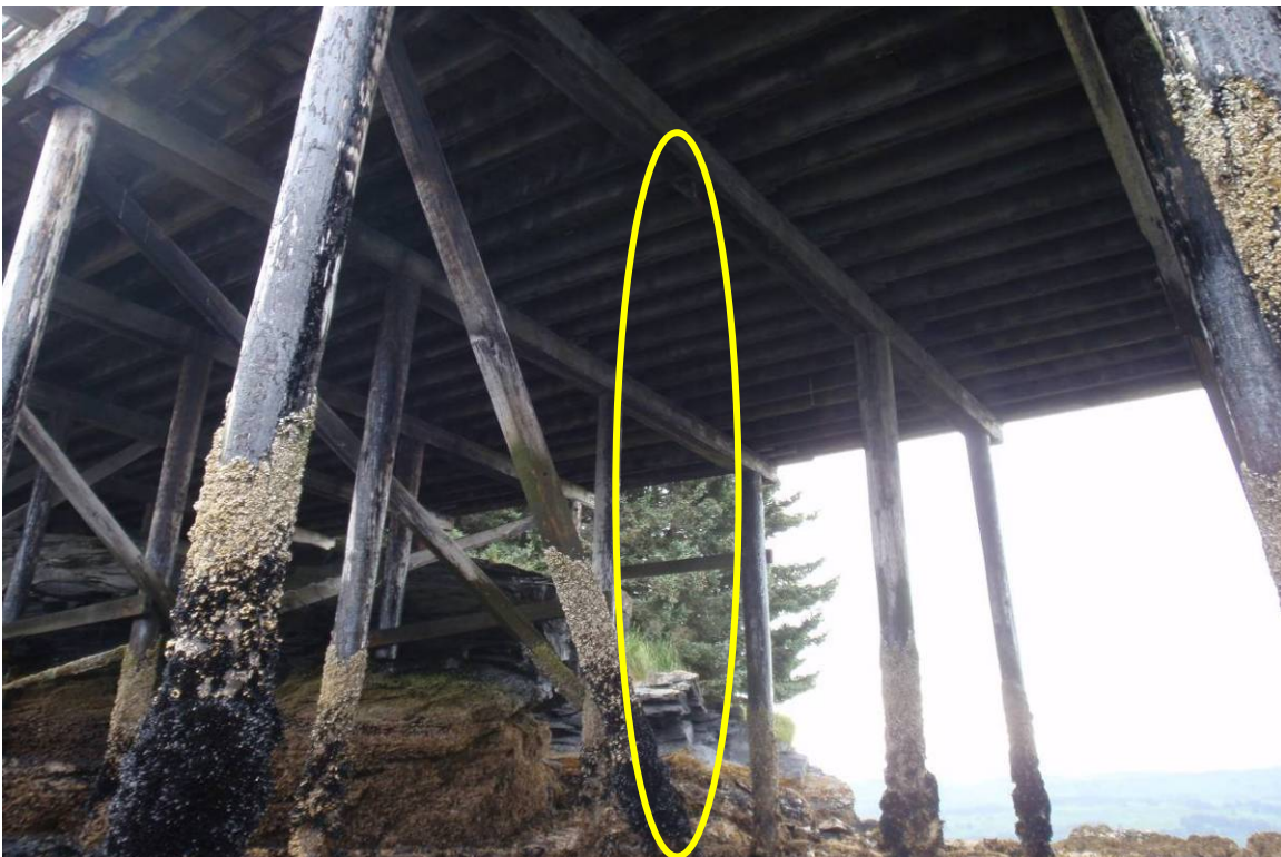
Photograph 8. Bent 10 – Pile C Missing
