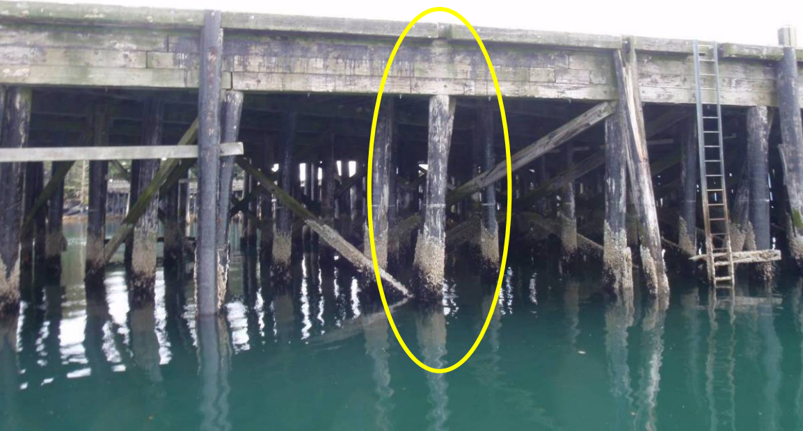
Photograph 13. Timber Fender O Missing
