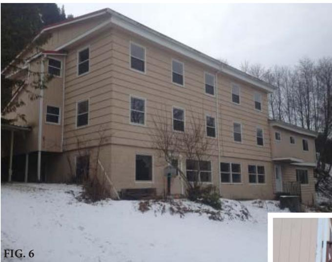
**Building:** The existing building consists of a daylight basement under a two story wood framed building. For clarity, they are referred to in this report as basement, main floor and second floor (fig. 6).
