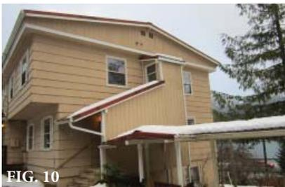
Exterior walls above the CMU are 2x4 studs with drywall and diagonal or plywood sheathing, with an exterior cladding of 3/8" re-sawn cedar plywood shingle panels. Interior face-of-stud walls are finished with drywall or plaster. In some locations there is no insulation (such as portion of the CMU walls). In other places we detected R11 fiberglass batt insulation. In no locations did we detect a vapor barrier.
