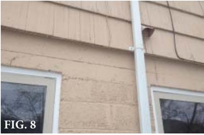
The basement consists of a slab on grade with 8" concrete masonry units (CMU) on the retaining walls (north, west and east walls) and 6" CMU in non retaining wall conditions (South and portions of west and east walls. The 6" CMU walls are topped with a 6"x16" cast in place concrete bond beam (fig. 8). It is unknown if the CMU is reinforced or not. The slab is covered with a wood floor consisting of wood furring under plywood. We did not detect water leaking in the CMU walls.
