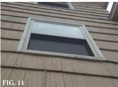
Windows are double hung vinyl replacement windows installed in the original openings. Exterior doors are insulated metal doors (fig. 11).
