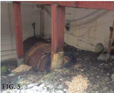
There is an abandoned oil tank, approximately 1,500 gallons under the elevated deck at the east end of the building. We have been told it holds approximately 40 gallons of old fuel (fig. 5).
