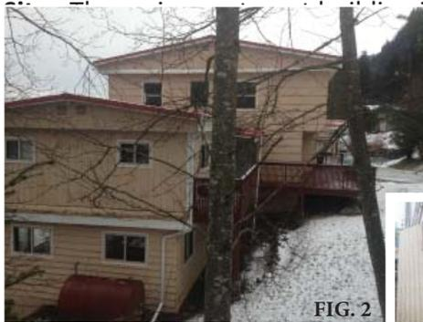
The building is located on a sloping site parallel to Glacier Highway, with the long axis running east-west and perpendicular to the slope (fig. 2). The sloping site necessitates the first floor being a daylight basement. The site appears to consist of unconsolidated overburden on a rocky substrate- a rock outcropping is visible under the Annex building (fig. 3).
