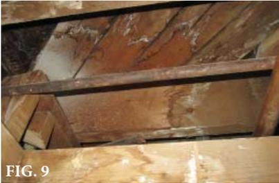
The floor framing above for the main floor consists of 2x12 at 16" (fig. 9). There are multiple layers of ceiling soffits apparently installed over the years attached below the floor framing reducing the floor to ceiling height to less than 7 feet. The second floor framing is similar to the main floor. Roof framing appears to be spaced 2x rafters installed at a 3:12 pitch installed over an original flat roof structure. It is topped with exposed fastener metal roofing (fig. 10).
