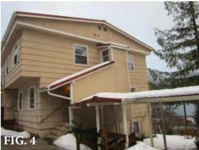
The building includes an elevated deck on the north side aligned with the sidewalk linking parking with the other site elements. The daylight basement has a doorway to grade on the south side. On the west side there is a doorway with steps leading up to the covered sidewalk connecting directly to the Adult Day Center. The adjacent grade is retained around the doorway area with rockery retaining walls (fig. 4).
