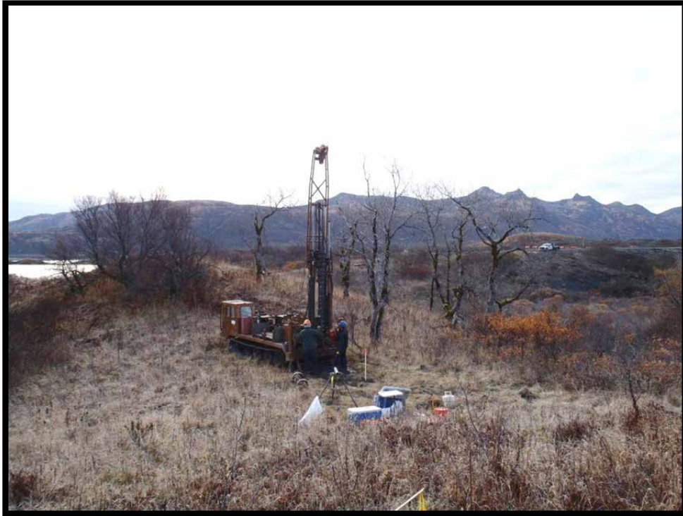
Test boring location RM12-07, as viewed from the north, 24 October 2012
