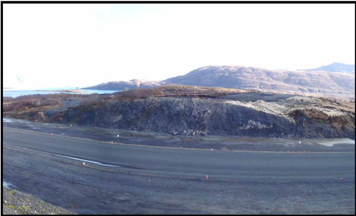
The existing southern runway rock cut, as viewed from the northwest, 26 October 2012
