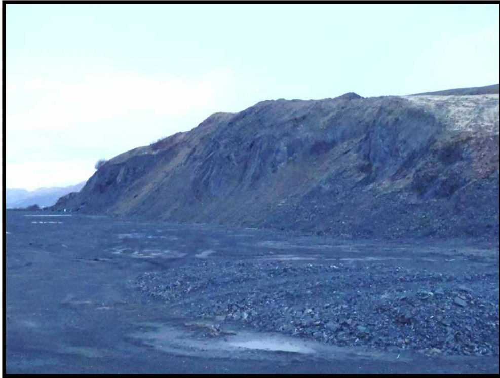
The existing northern runway rock cut, as viewed from the east, 26 October 2012
