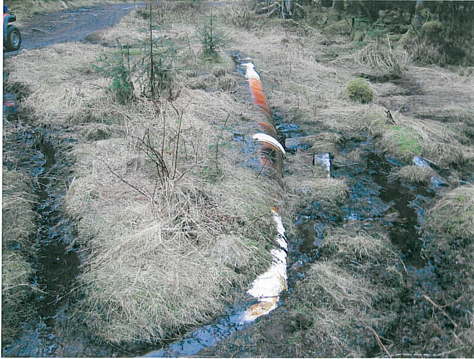
Picture #3 – Exposed Transmission Pipe
