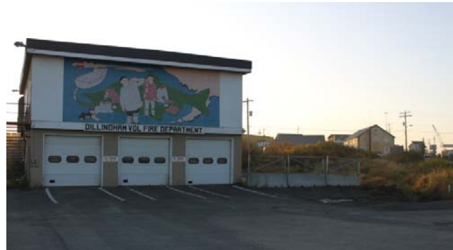
Figure 5 Dillingham Fire Hall bays are too short for new equipment.
