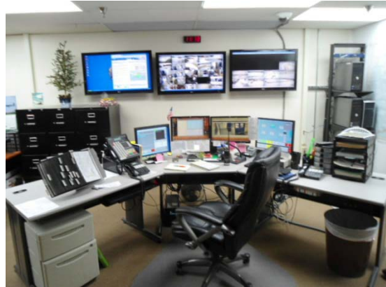
Figure 9 Dillingham Police Dispatch Center
