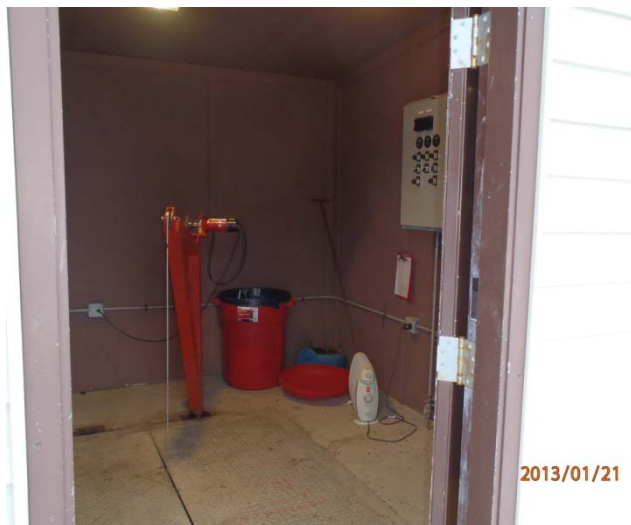
Figure 8 Lift Station with multiple mechanical, structural and electrical defects
