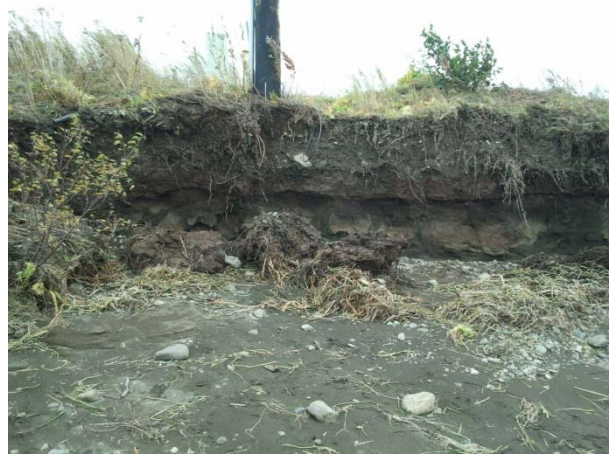
Figure 14 Erosion of East bank in harbor exposes utilities
