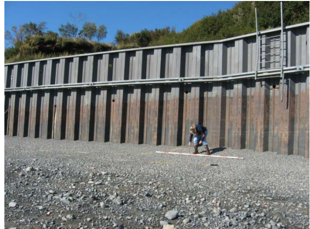
Figure 16 Snag Point Bulkhead
