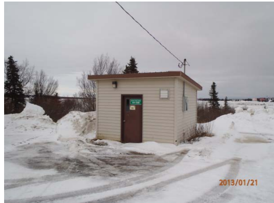
Figure 7 Smalls Lift Station
