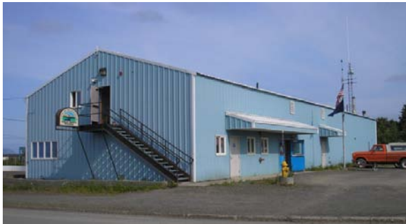
Figure 6 Public Safety Building
