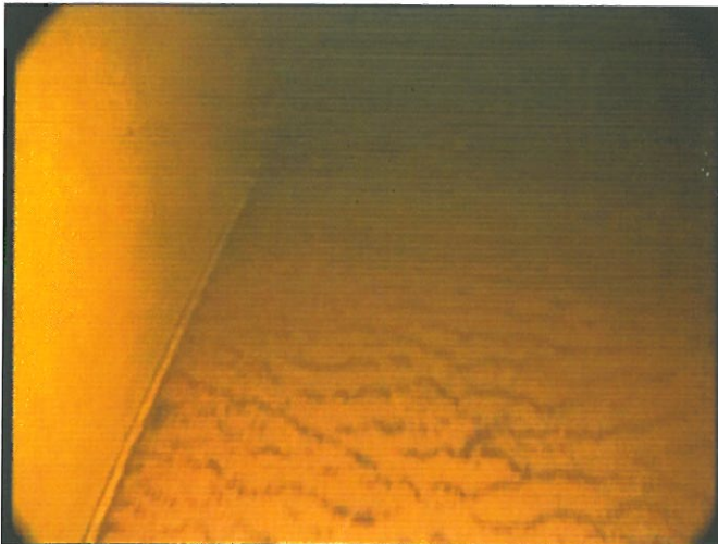
Minor dusting of sediment on tank floor (Time 27:29)
