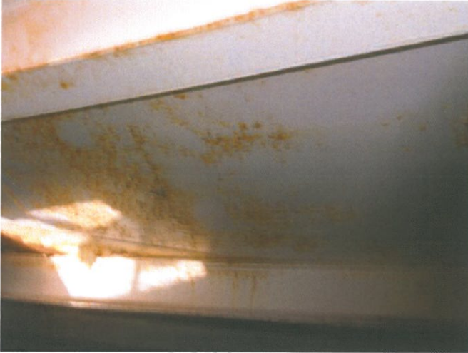
Pinpoint corrosion on interior roof plate
