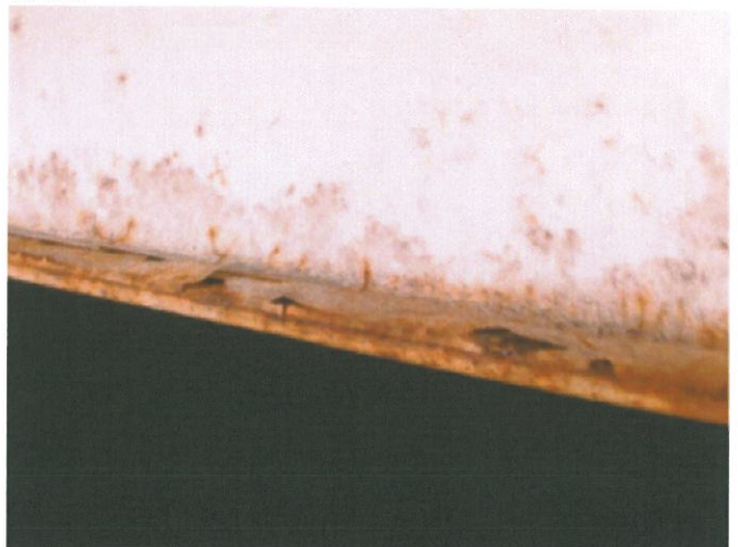
Corrosion and coating failure on roof support beam
