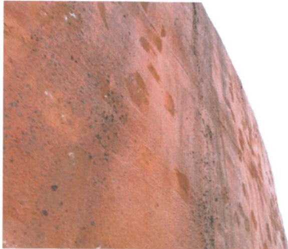
Upper shell insulation has slight deterioration
