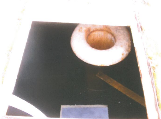
36-inch square roof hatch with edge corrosion on sanitary curb
