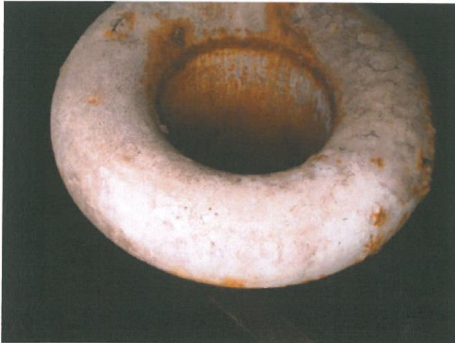
Overflow pipe with cone top
