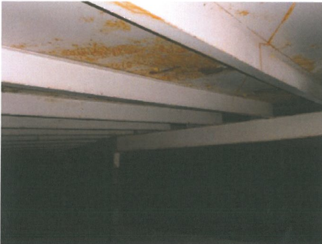
Pinpoint corrosion on interior roof plate
