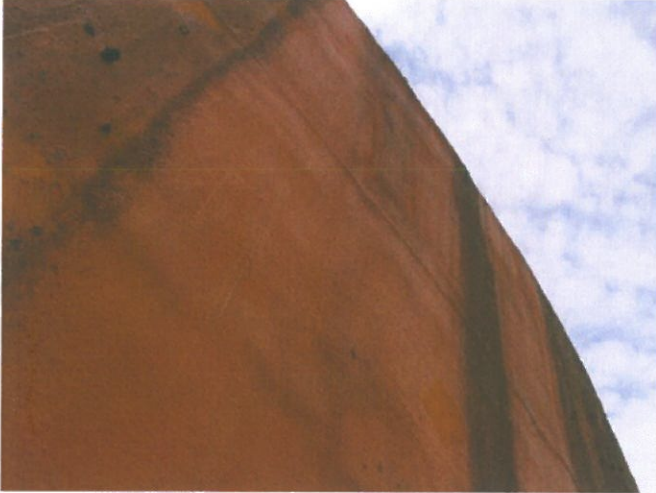
Upper shell insulation in good condition
