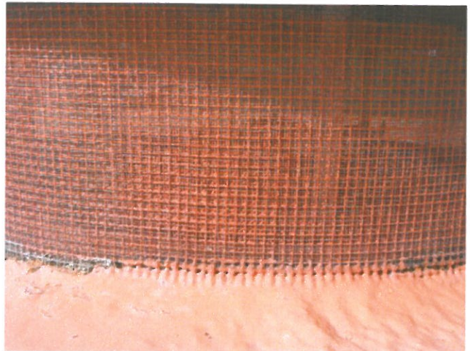
Coarse and fine mesh screen on roof vent.
