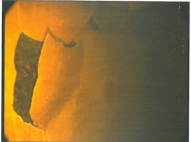
Large area of coating failure and surface corrosion on upper shell plate (Time 47:47)
