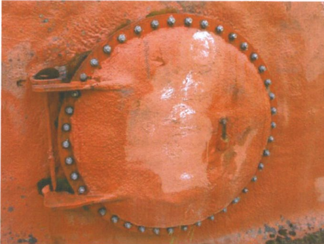
36-inch shell manway
