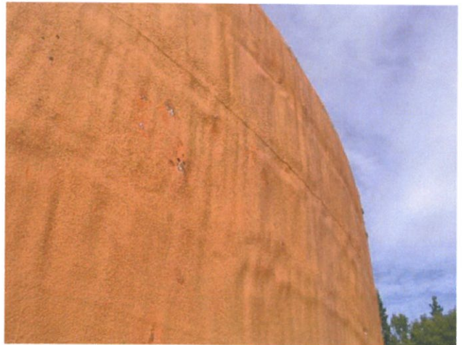
Upper shell insulation with rock damage
