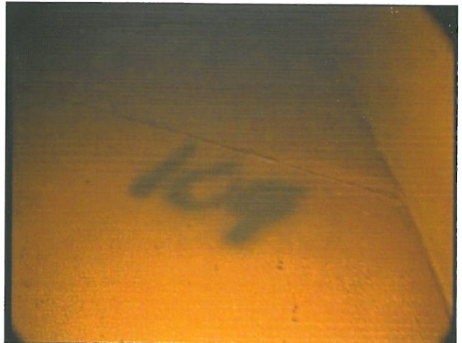
Light staining on floor plates (Time 36:01)
