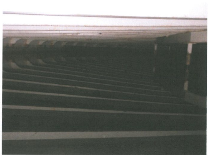
Interior roof support beams with minor edge corrosion
