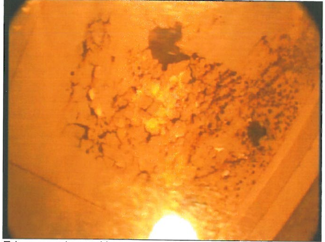
Edge corrosion and large area of coating failure on roof plates (Time 2:53)
