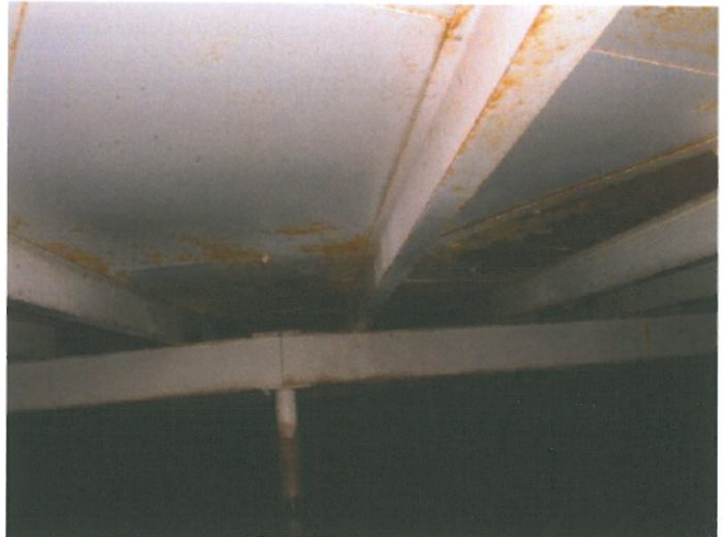
Pinpoint and edge corrosion on interior roof plates and beams
