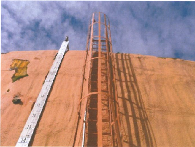
Exterior shell ladder with safety cage
