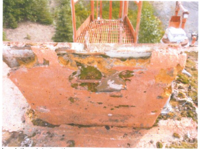
Insulation deterioration on roof hatch lip
