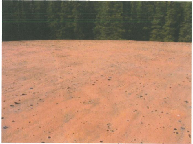
Insulation deterioration on exterior roof
