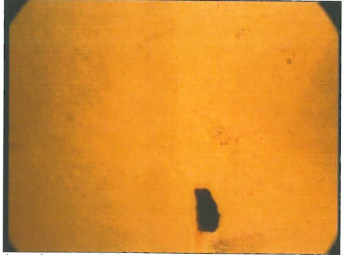
Area of coating missing with surface corrosion (Time 9:00)
