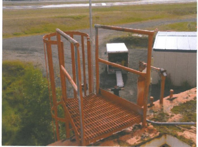
DP#10 Railing system adjacent to roof hatch
