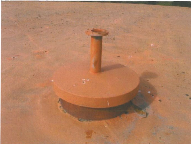
Center roof vent cap
