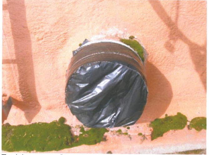
Trash bag on overflow discharge
