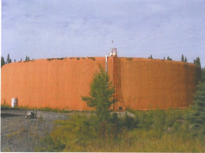
Overall view of tank
