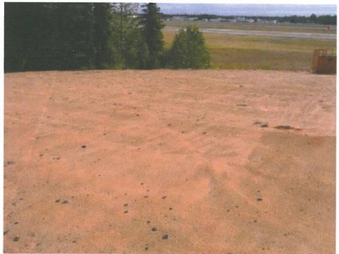
Insulation deterioration on exterior roof plates
