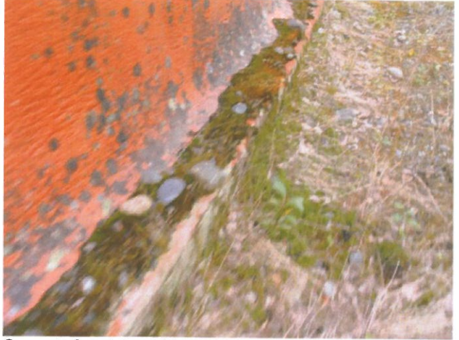
Concrete foundation with minor spalling
