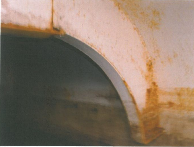
Pinpoint and edge corrosion on roof support bracket
