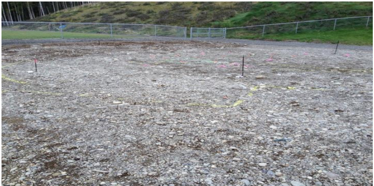
Laying out the location of the playground equipment.
