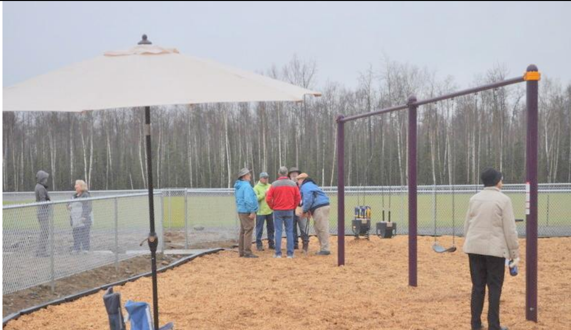
View of fencing installed to separate soccer field and playground areas.
