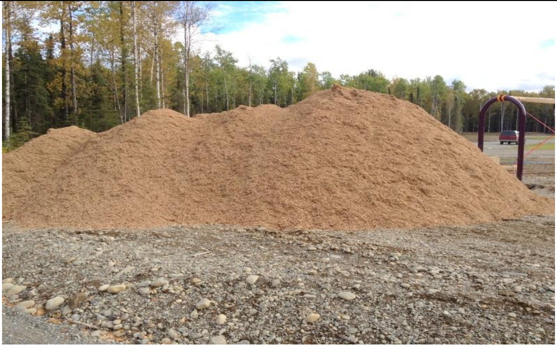
Engineered Wood Fiber safety surfacing arrives from Valley Sawmill
