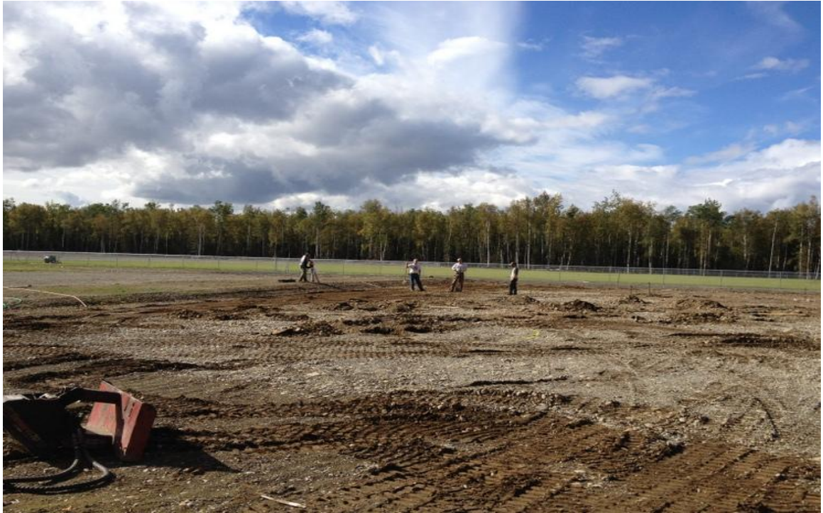
Playground installation begins with shooting the corners and leveling the site
