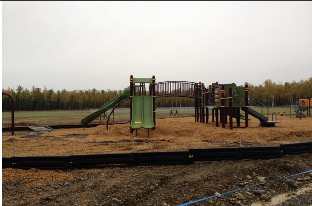
Installing the safety surfacing
