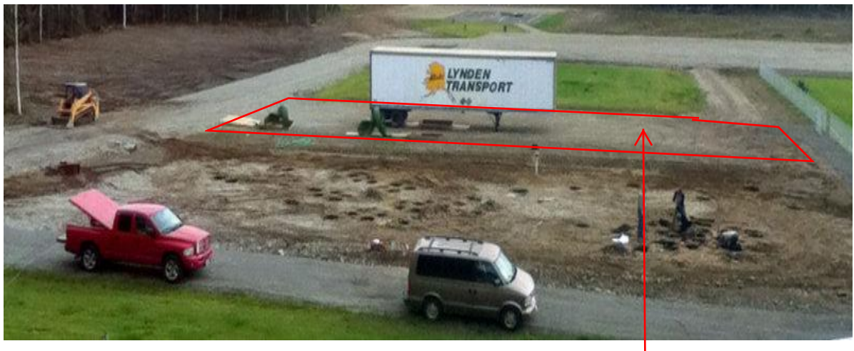
The Lynden Transport container is where the parking lot for playground is located. This area needs to be paved to allow for accessible access.
