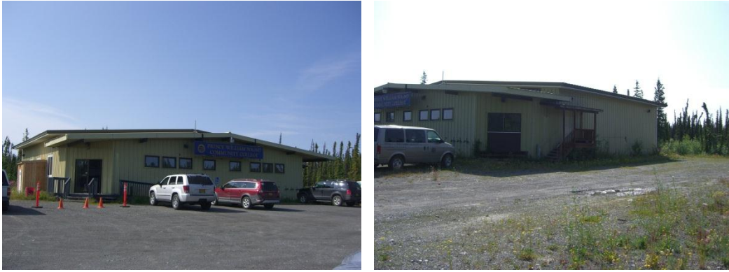
Figure 5: Left: Face of Prince William Sound Community College. Right: East side of the facility, where the biomass boiler facility would be positioned.
