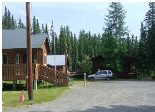
Figure 6: Cluster 1: from Left to Right: New Admin, Rec, and Old Admin Building. Truck access to proposed boiler facility is pictured on the right.
