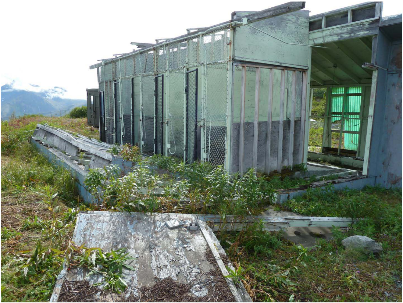
Dog Kennels heavily damaged by weather and time. FONSS took on restoration of the Kennels as an additional task.
