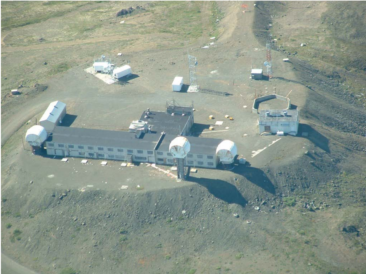
Upper Site Summit before demolition of the Battery Building. Roof leaks caused such extensive damage that JBER determined that demolition of this building (which served as both Dormitory, and Headquarters) was necessary.
