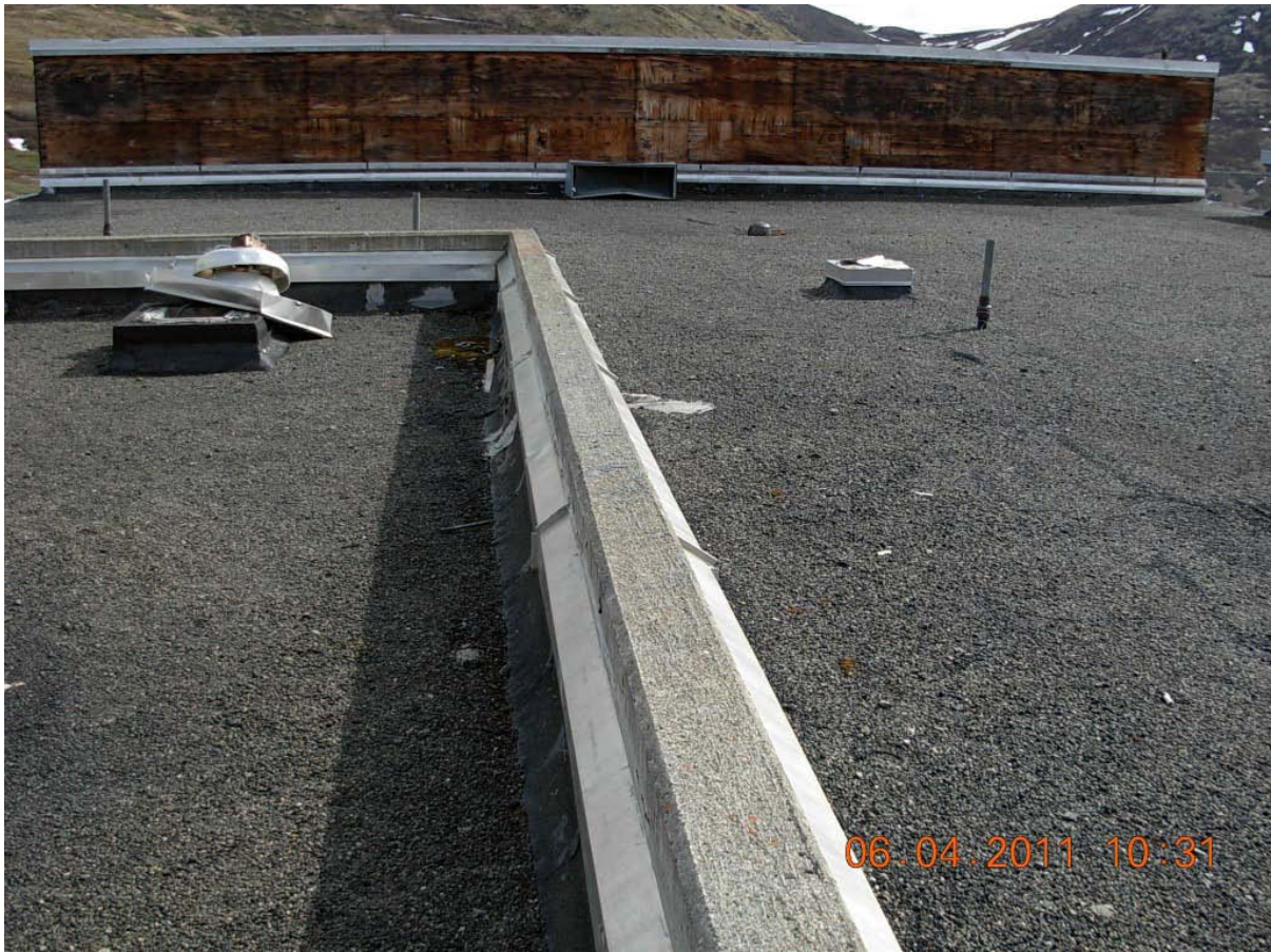
Roof over Launch Control Building, before re-roofing.
