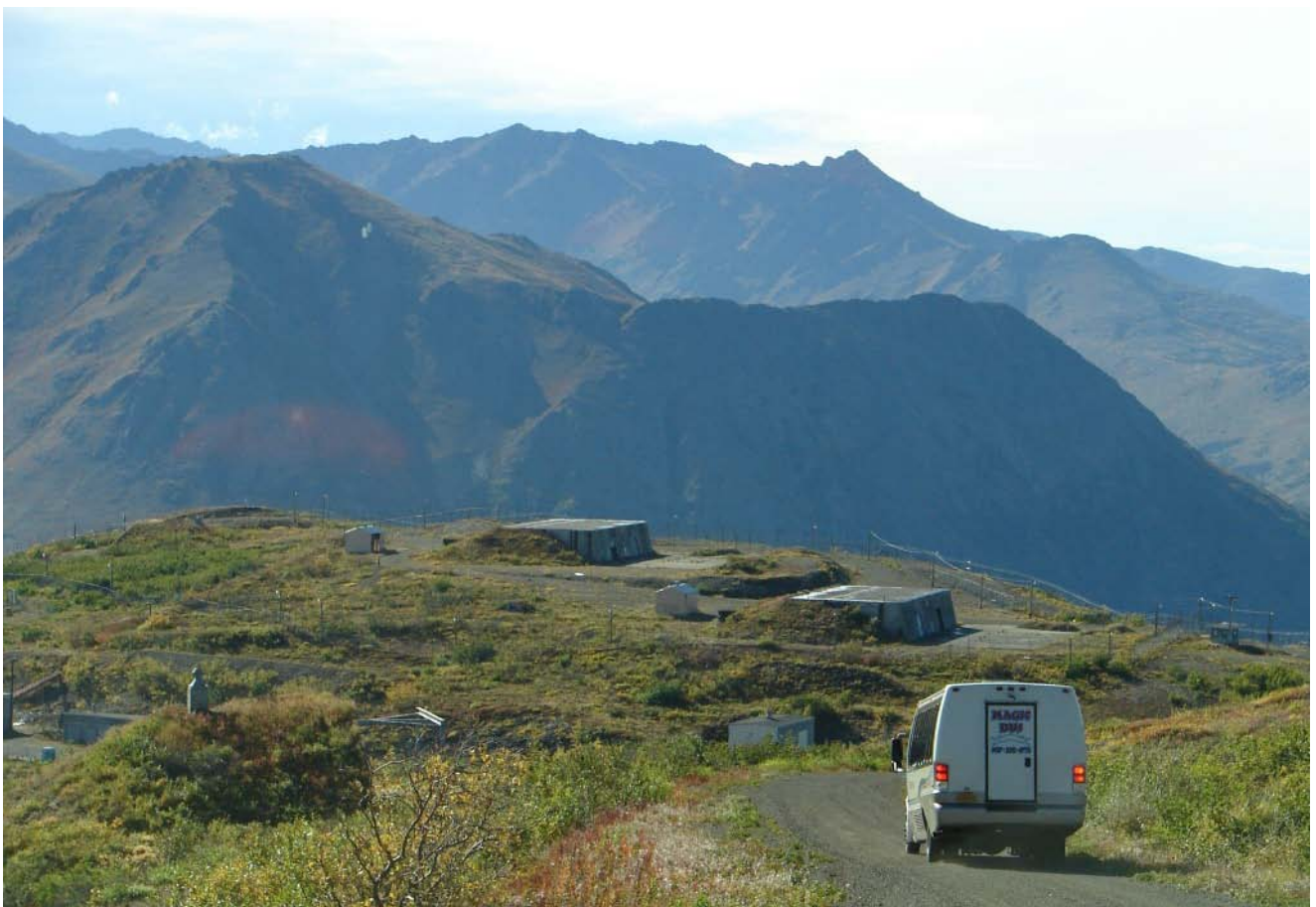
FONSS Tour Bus heading to Lower Site Summit. Note re-sited Missile Maintenance Building just left of Bus.
