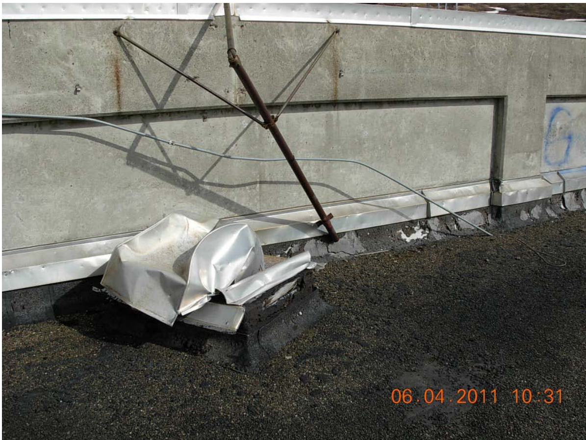
Badly deteriorated roof over Missile Control Van Room of Launch Control (Roof D of this Funding Request)
