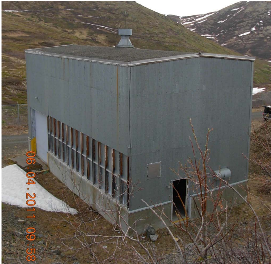
Missile Maintenance Building, before siding repairs.
