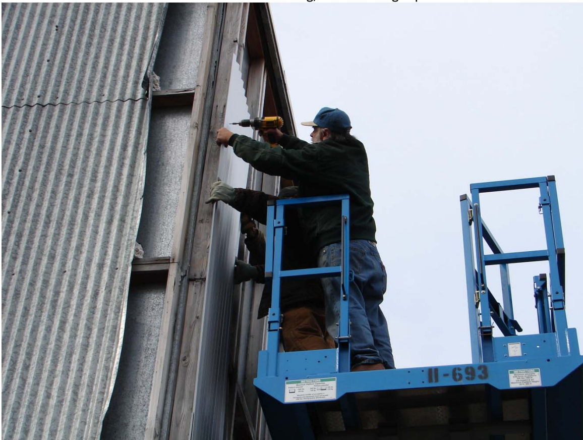
Siding Repairs on Missile Maintenance, from donated man-lift.
