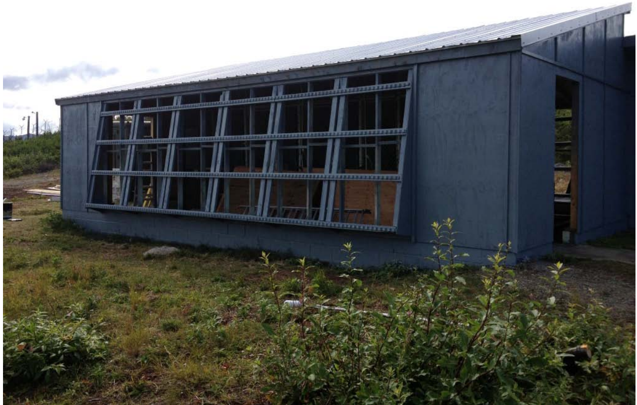
Dog Kennels during re-construction and restoration. The “window” elements are original, dug out of the tundra Alaska Association for Historic Preservation CAPSIS Nike Site Summit Roof Repairs Page 7 of 11
