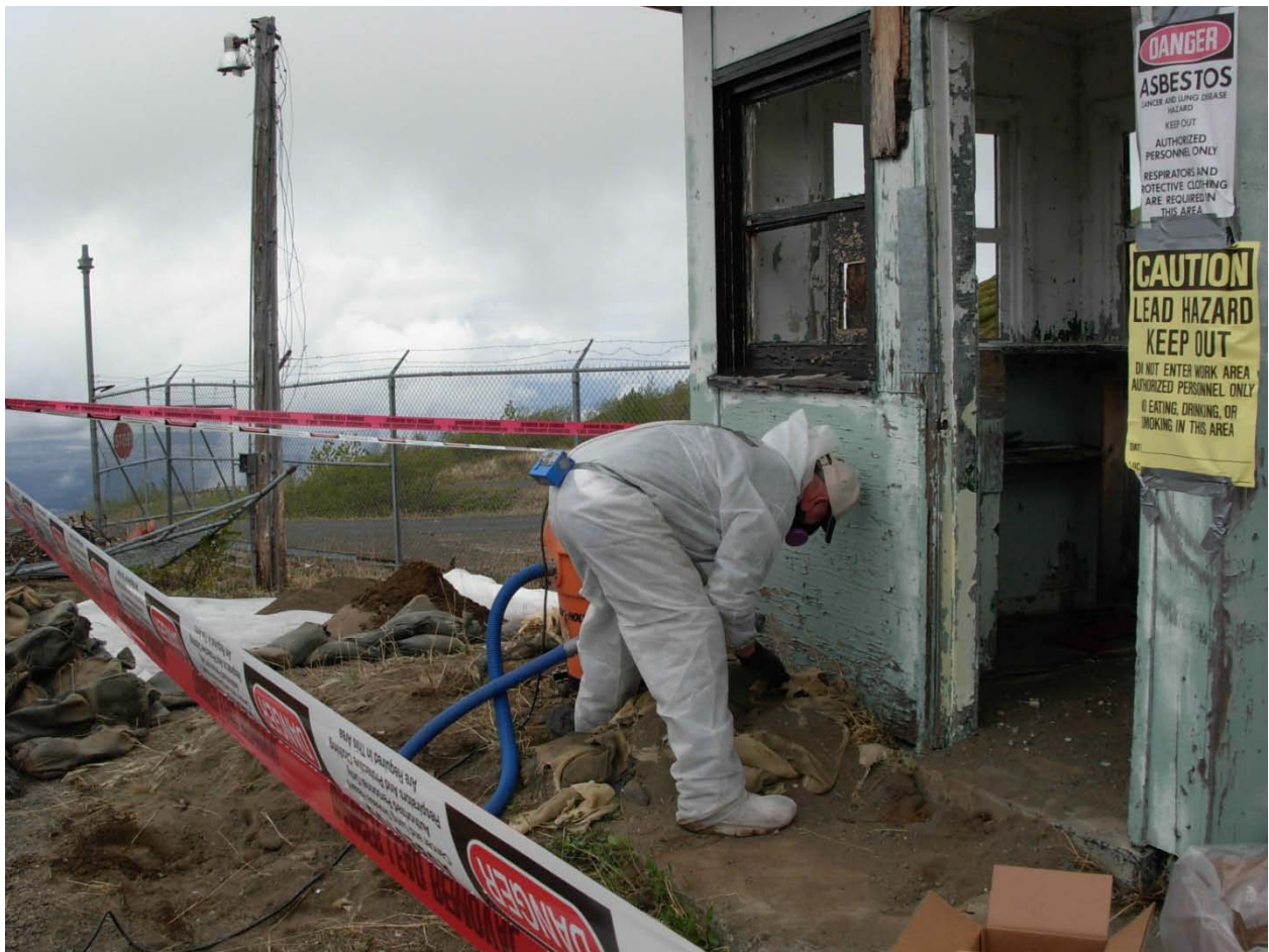
Abatement work at Sentry Station 1
