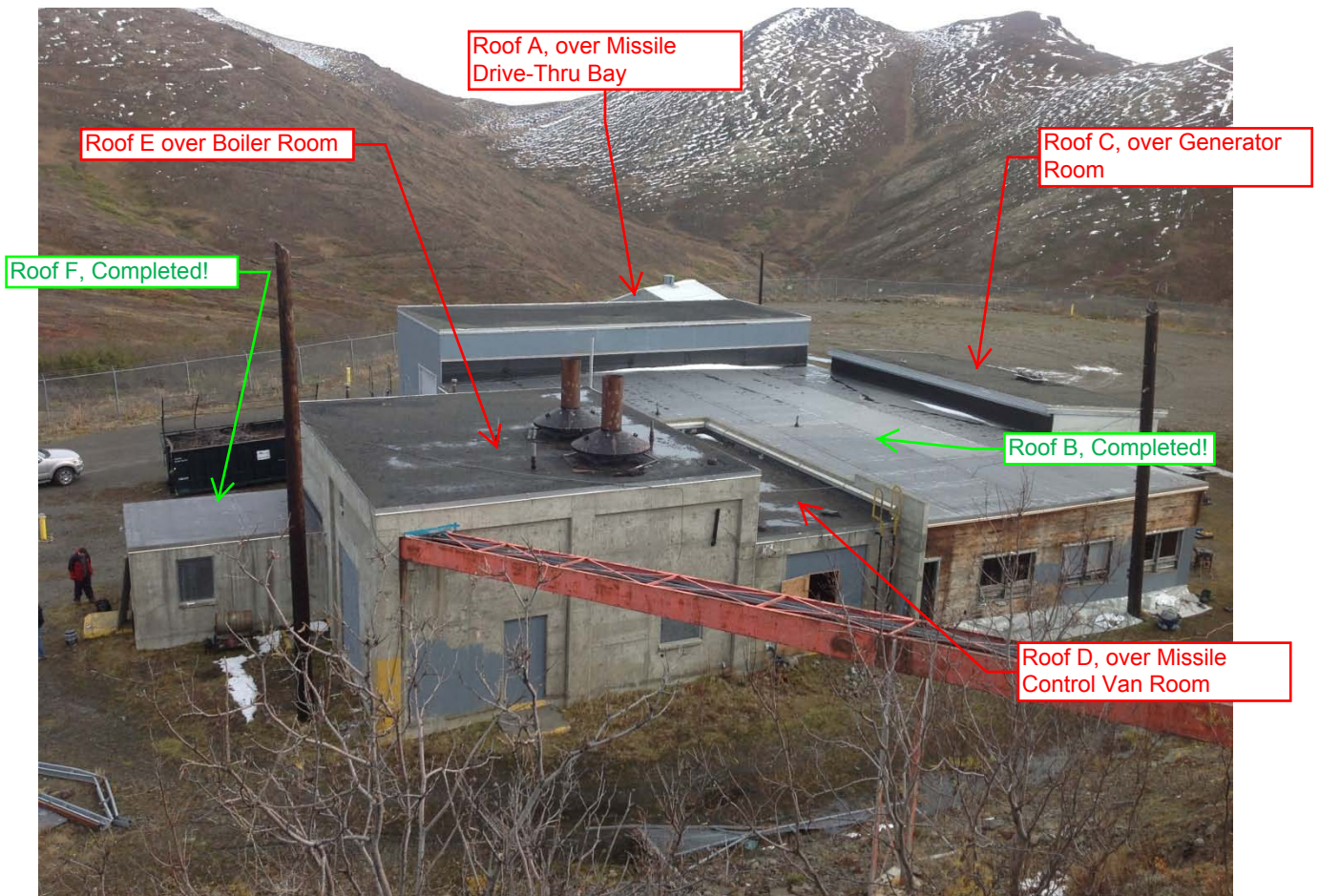
Launch Control Building in 2013, Completed roofing, and roof areas that are part of this Funding Request.
