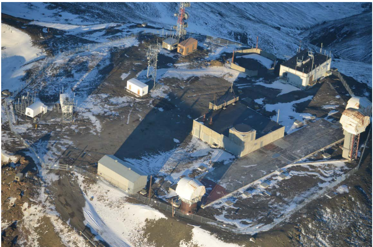
Upper Site Summit, after Demolition of the Battery Building
