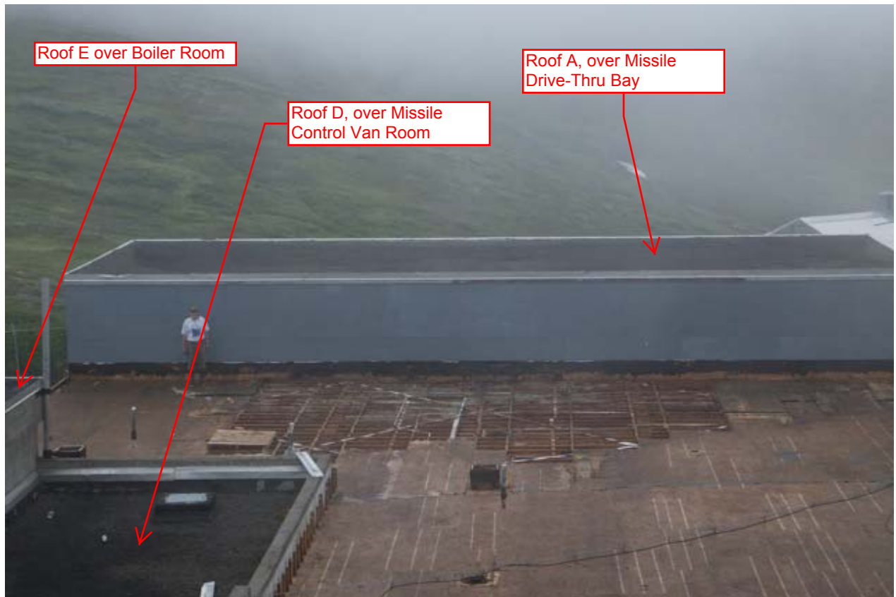
Removing rotted wood roof deck over Launch Control Bldg. All 3 black surfaced roofs are part of this Funding Request
