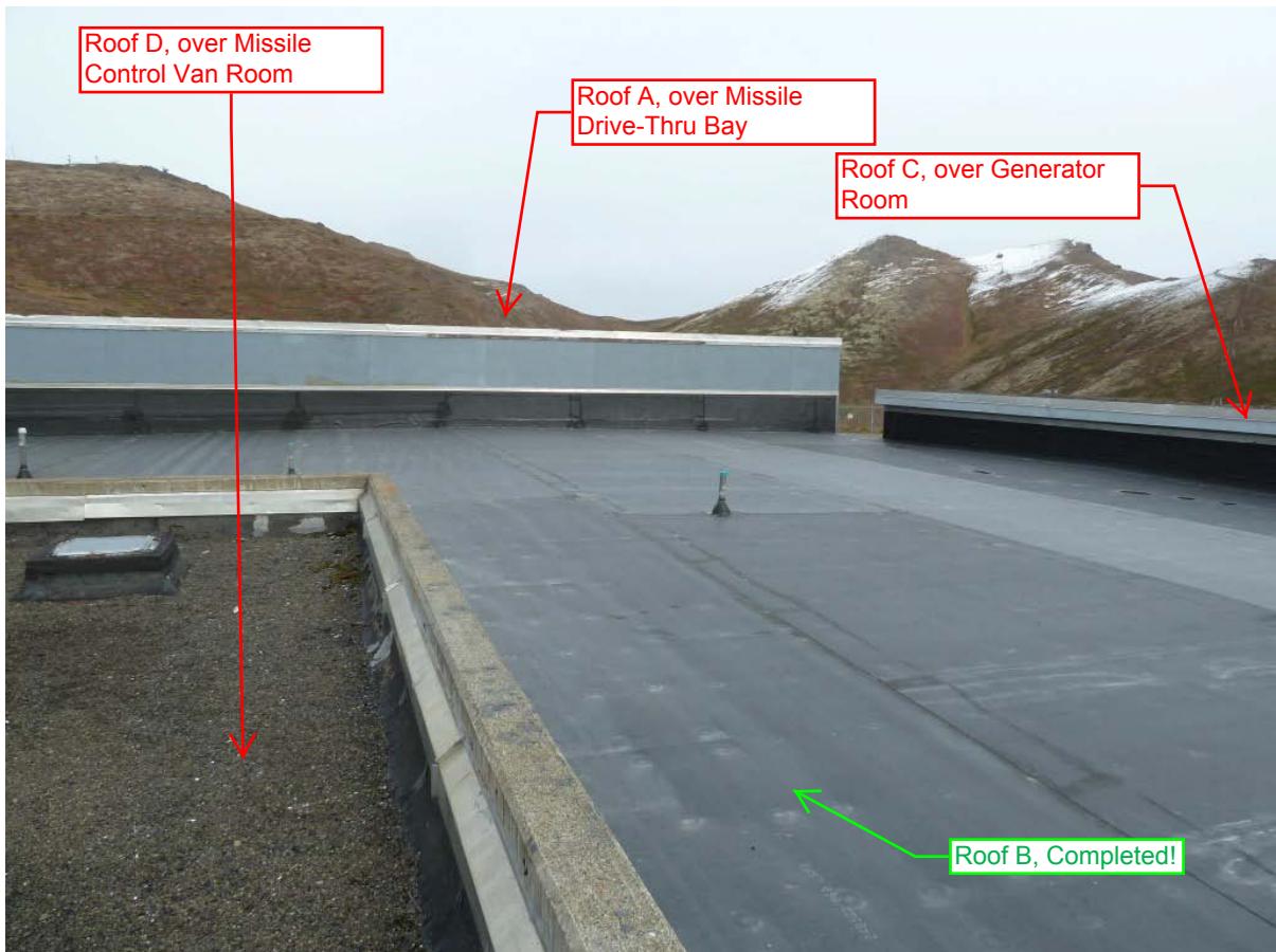
Roof over Launch Control, after. Roof to left is Roof D, over the launch control van, part of this Funding Request.
