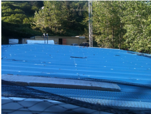
Metal roof deck.
