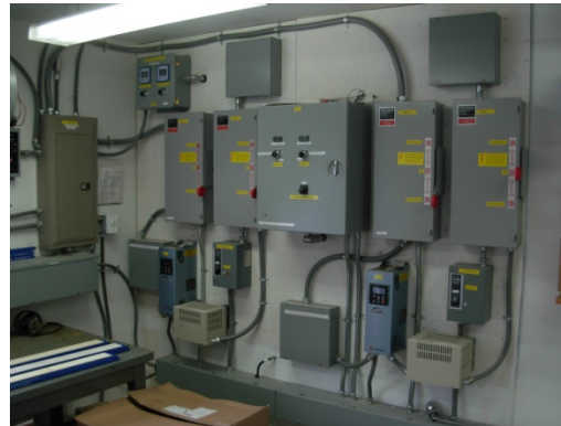
Compressor/Oxygen Building Panel B and Well Pump Controls
