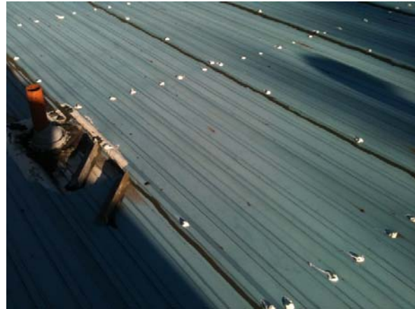
Sealant at metal fasteners.
