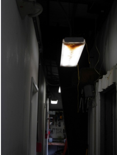
Lighting in corridor
