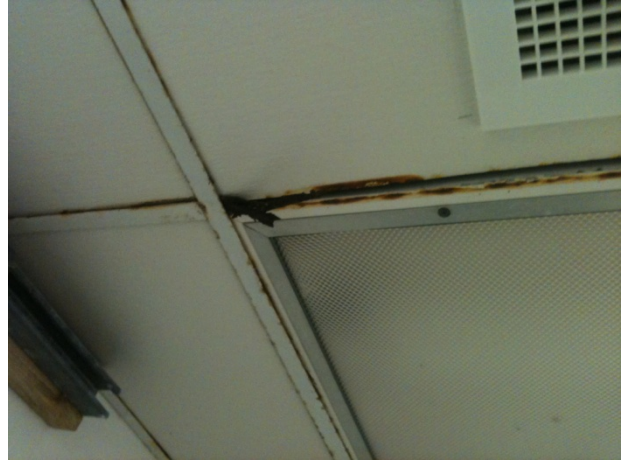
Water damaged ceiling tiles.
