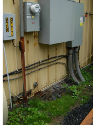
Service meter and main disconnect
