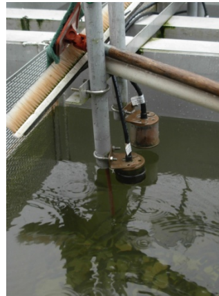
Raceway level switches
