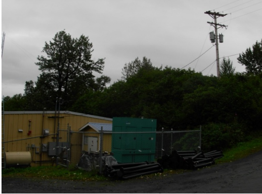
Service equipment and generator
