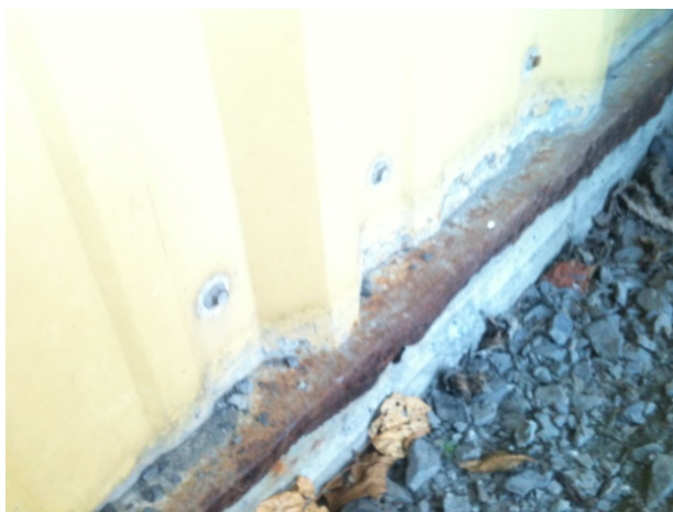
Above: Deteriorated sill flashing
