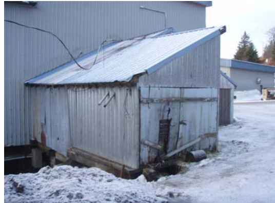
Deteriorated siding
