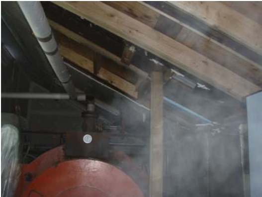
Suspicious roof framing in east portion of roof
