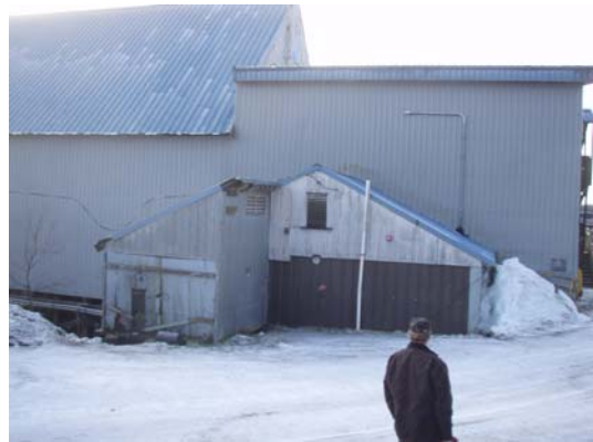
Exterior from north side
