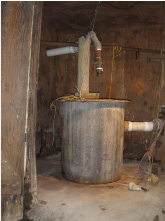
Sewage pump wet well- note float controls on floor
