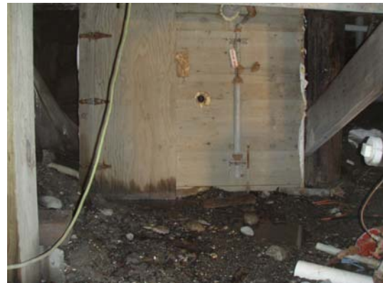
Exterior of sprinkler riser room
