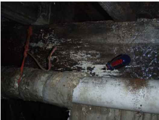
Rotten pile cap penetrated by screwdriver
