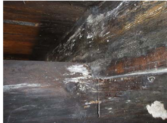
Crushed joist, fungus on joist and cap
