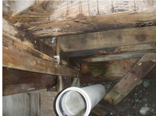
Foundation drain daylighting into crawl space
