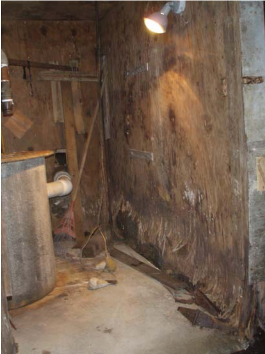
Failed sheathing at sewage pump station room
