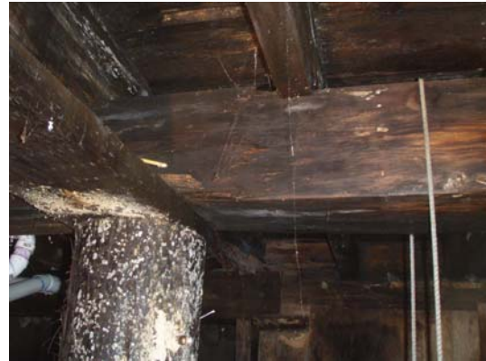
Cracked and crushed pile cap
