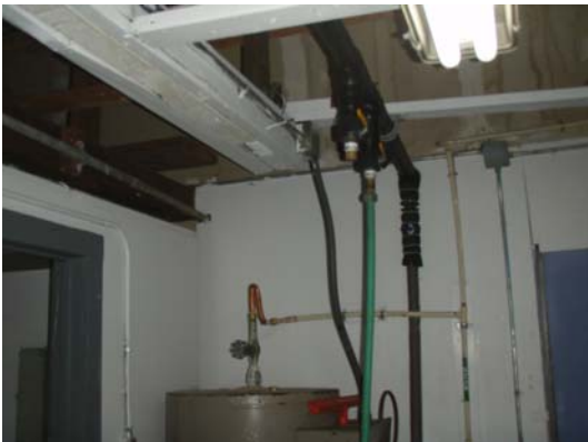
Severed roof truss
