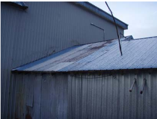
Deteriorated roofing east side
