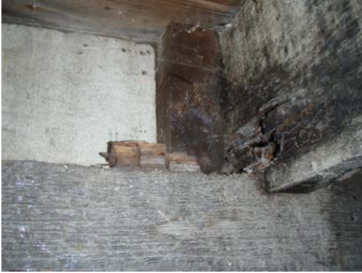
Rotten end of floor joist – Note crushing.
