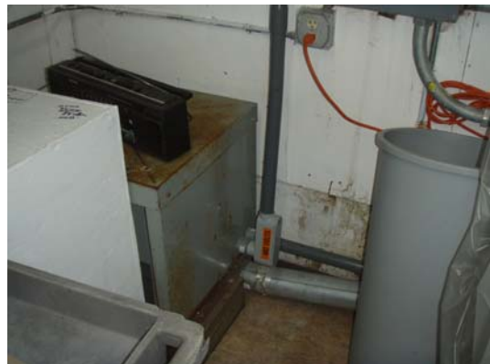
Transformer without proper clearance
