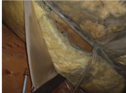
Damaged vapor barrier and insulation
