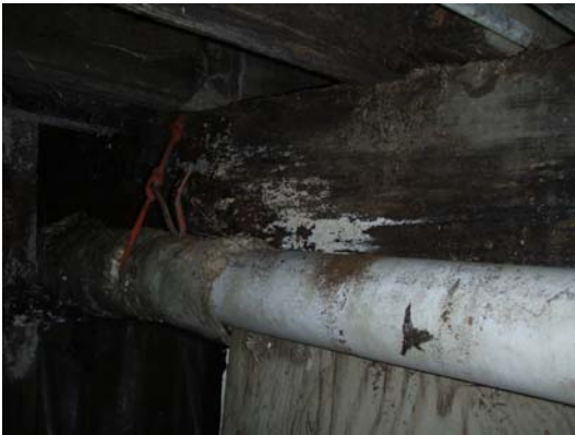
Fungus on pile cap
