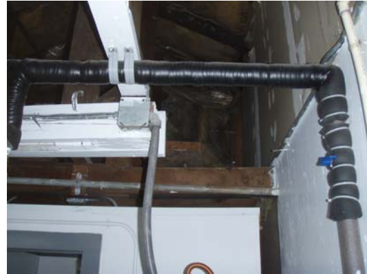
Another view of severed roof truss
