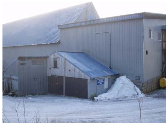
Exterior from north west
