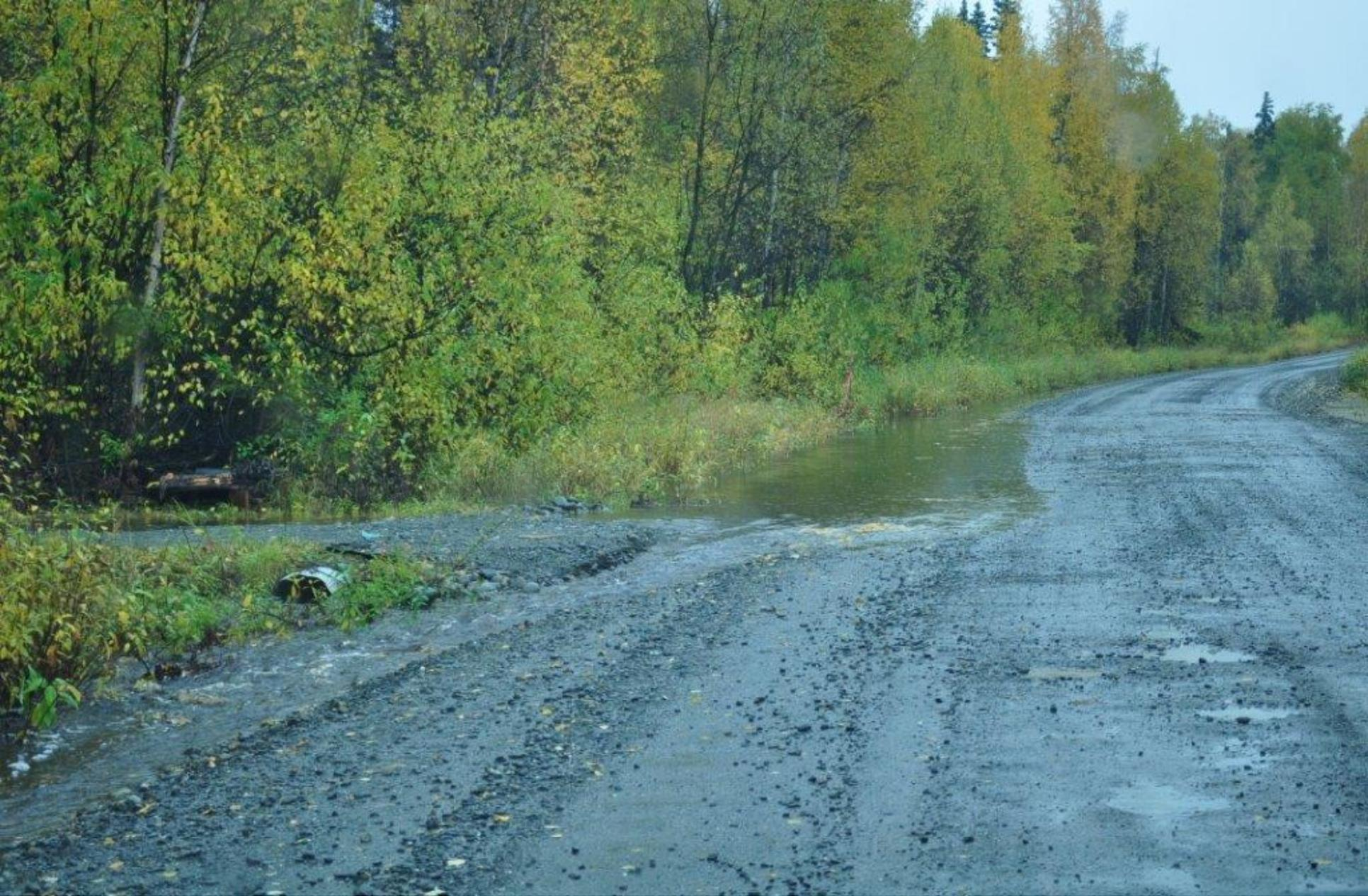
Oilwell Road approximately mile 2 during October 2012. Oilwell Road floods during break-up and seasonal heavy rain. Poor drainage and road elevation result in swamps flowing onto the road for up to  $\frac{1}{2}$  mile lengths at full road width making travel impossible for up to 400 residents.
