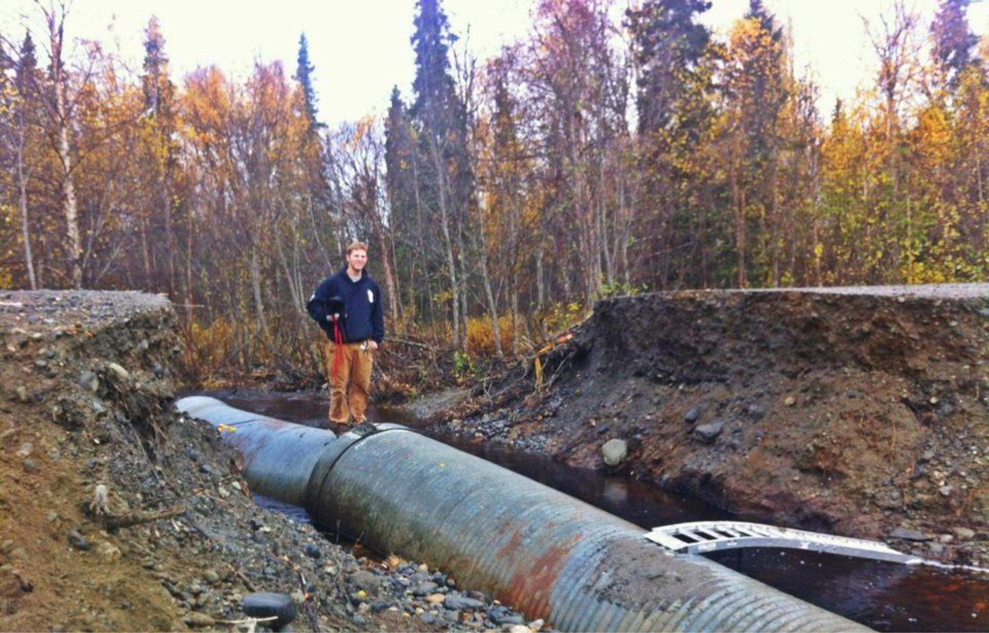
September 2009. Oilwell Road residents added a loading ramp in the foreground to allow foot traffic to homes. Road failure is a common occurrence due to improper drainage and poor construction.
