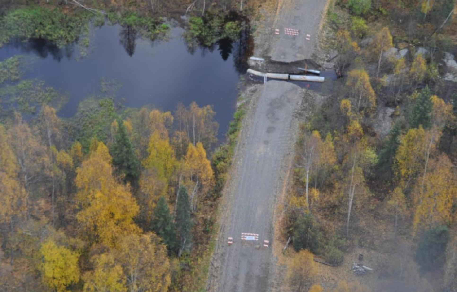
Aerial view of Oilwell Road in September 2009. Improperly constructed drainage systems along the road result in road failure during heavy rains and rapid melt off events leaving residents stranded and cut off from emergency services.
