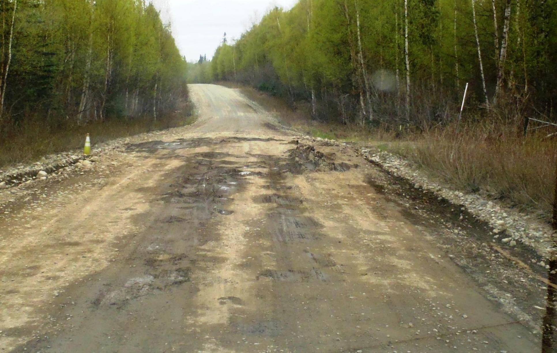
Another of the more than 100 locations where Oilwell Road is failing due to poor road materials and drainage problems. This photograph was taken as part of a 2011 survey of conditions.
