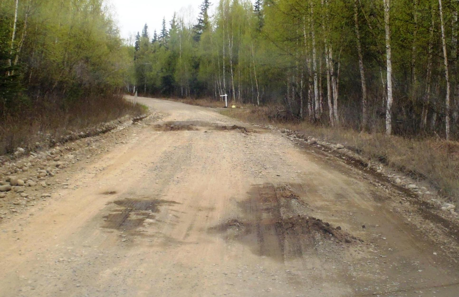
Oilwell Road in May 2011. At over 100 locations on the first six miles the road is failing due to improper drainage and underlying frost susceptible materials which percolate to the surface as vehicles compress the soil.
