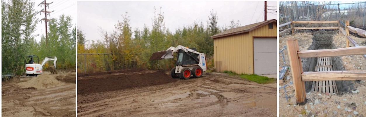
Figure STEAM 10. Facilities Services creates the University Park Forest Education Outreach Center on University Ave. near campus. On left: excavating the trench, Center: building transplant beds; on right: the finished 18'x4'x4' trench, ready to receive overwintering tree seedlings and insulated cover.
