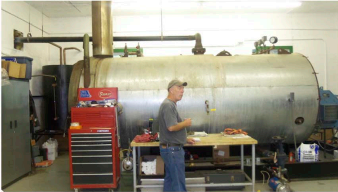
Figure STEAM 24. Harold Torre in front of his boiler. Franklin County, VT.
