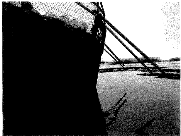
Photo 2: Leaning sheet pile wall.
