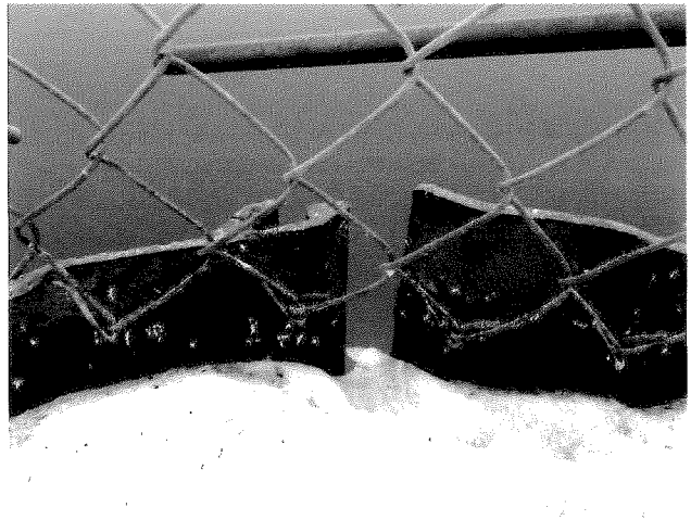
Photo 4: Separation at wall seam.
