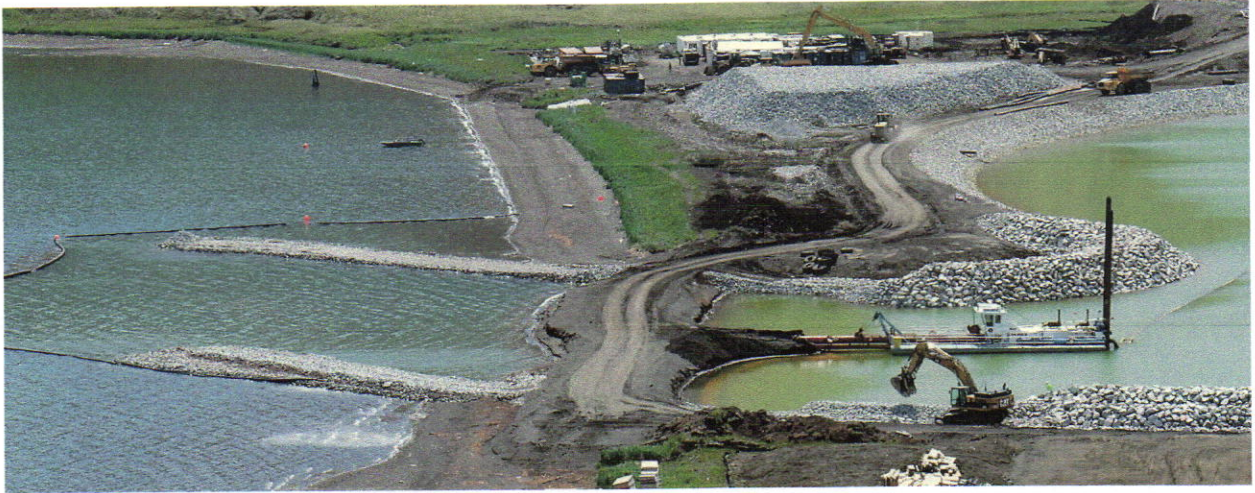
Construction of the Akutan Harbor – July 2012
