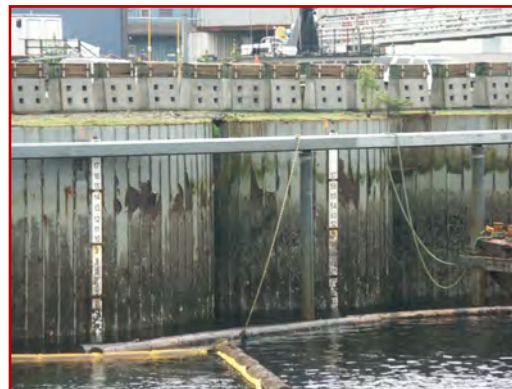
Sheet Pile Ring Cells
