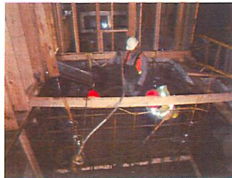
Journeyman Floyd Frank teaching the 2 apprentices how to pour concrete
