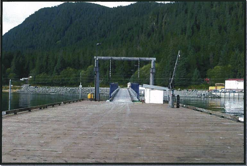
Juneau Drive Down Dock
