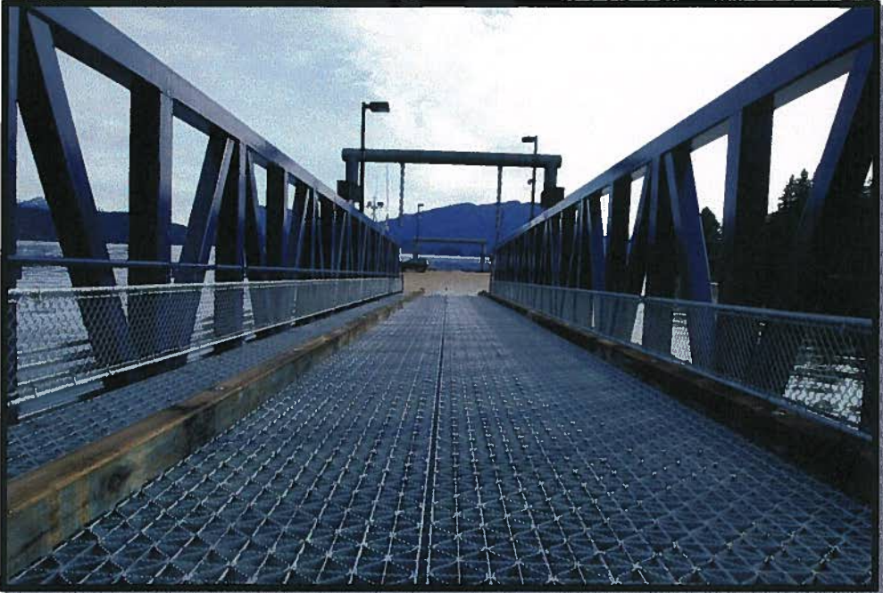
Juneau Drive Down Dock
