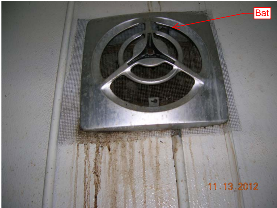
Vent with bat behind the screen
