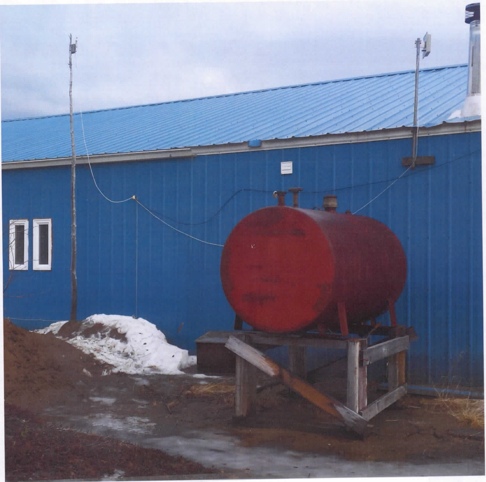
Need larger and additional windows to allow more sunlight in, in order to reduce the amount of energy being use.
