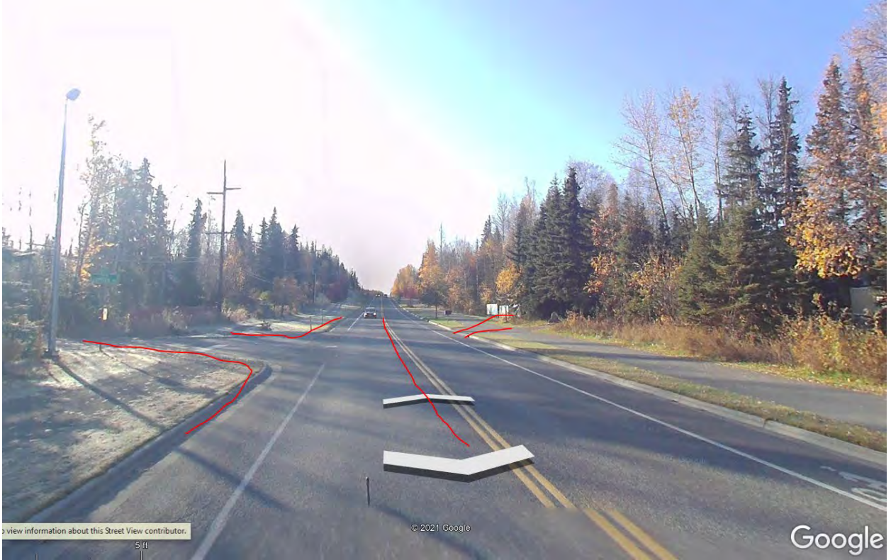
Elmore and Jupiter, Driveway close to 84 th Ave, South Leg, view South from 84 th
