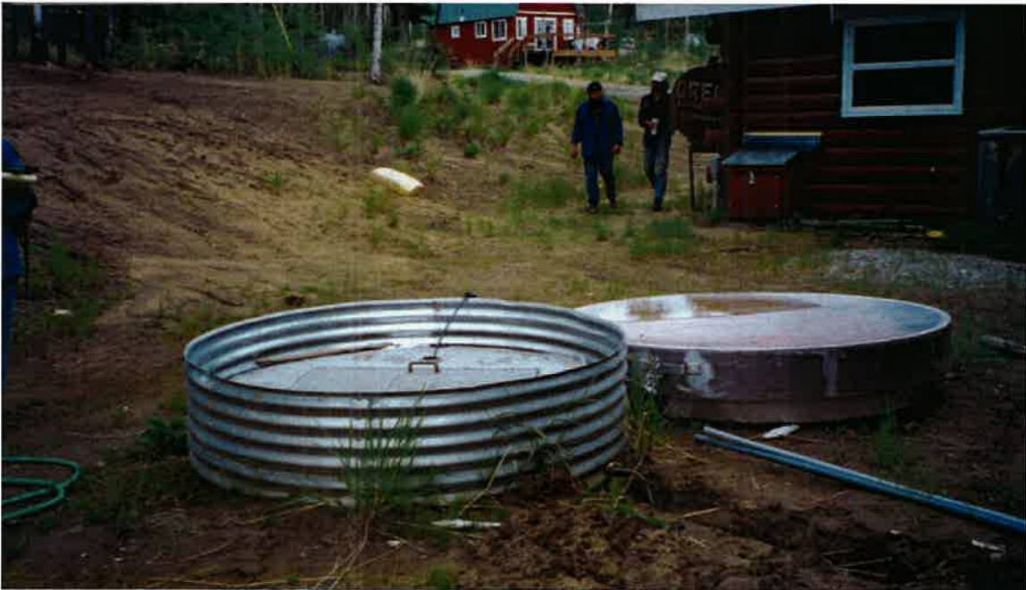
Photo 28. Lift station cover, 6/15/00.
